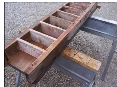
Figure 2. The assembled form on sawhorses
